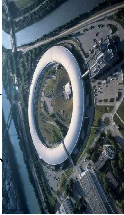
ESRF Synchrotron, Grenoble
